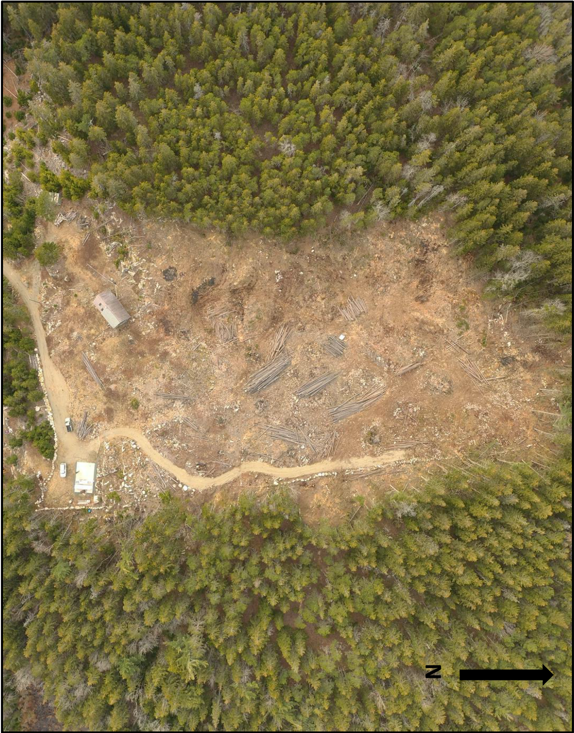
Fig. 3 Coomb's Mountain solar site August, 2020. Concrete pad in SE corner is approximately 40'x20.'
